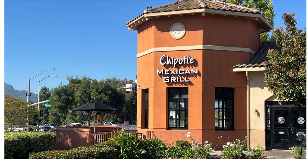
02 – Chipotle Sign Facing 101 Freeway
