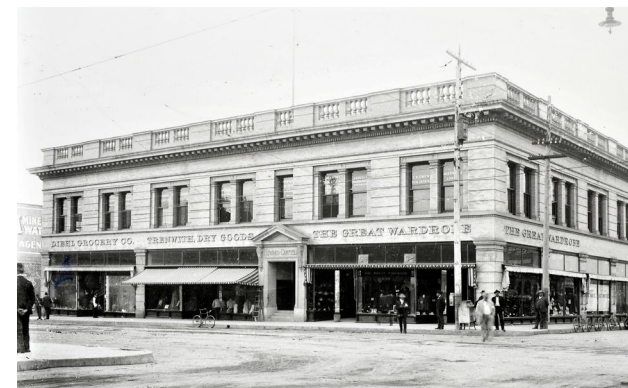
02 – Historical photo of the Howard Canfield Building.
