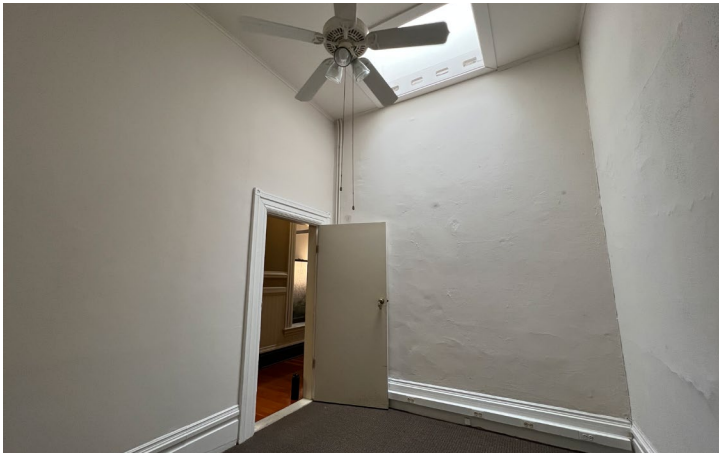
04 – Suite 229 interior with skylight.
