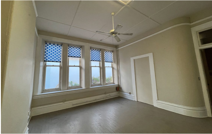
02 – Suite 250 Interior Pre-Renovation.
