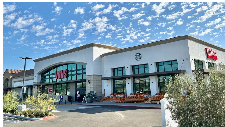
01 – Newly constructed 63,272 SF Vons
