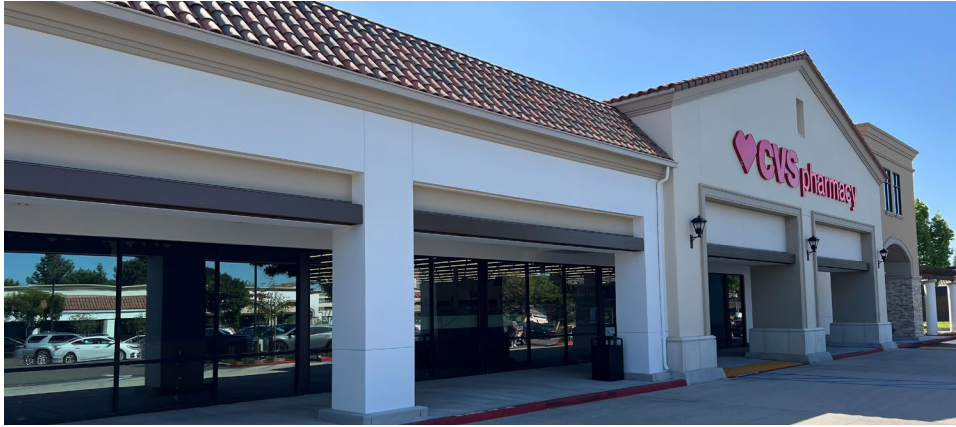
02 – 23,989 SF CVS with Full Façade Refresh
