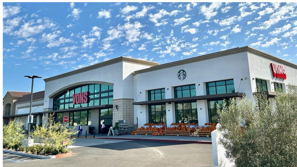
01 – Newly constructed 63,272 SF Vons
